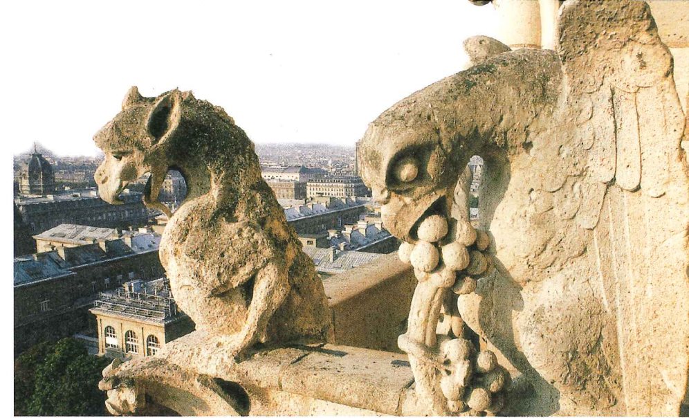
FIGURE 4 Effects of Chemical Weathering Acid rain chemically weathered these stone gargoyles on the cathedral of Notre Dame in Paris, France.
